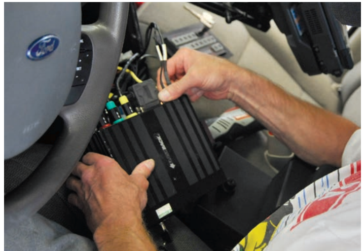
A telecom employee installing a Wyolink radio system in a WYDOT vehicle.
