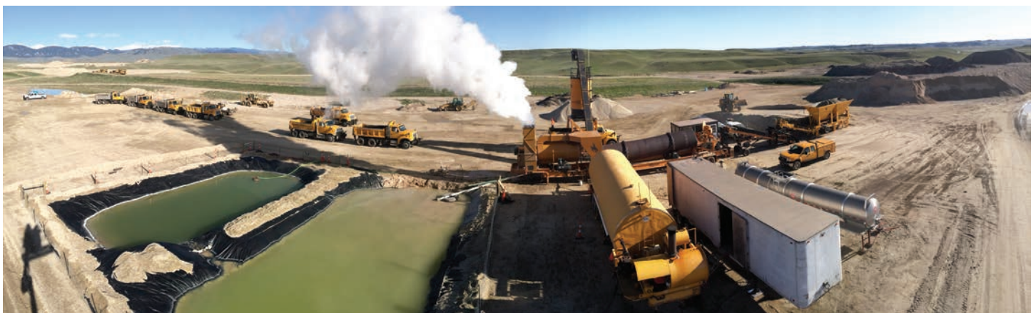
The District 2 hot mix plant in production just east of Guernsey.
