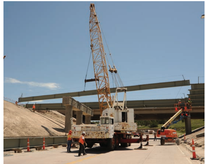
Bridge girders being placed in Pine Bluffs.
